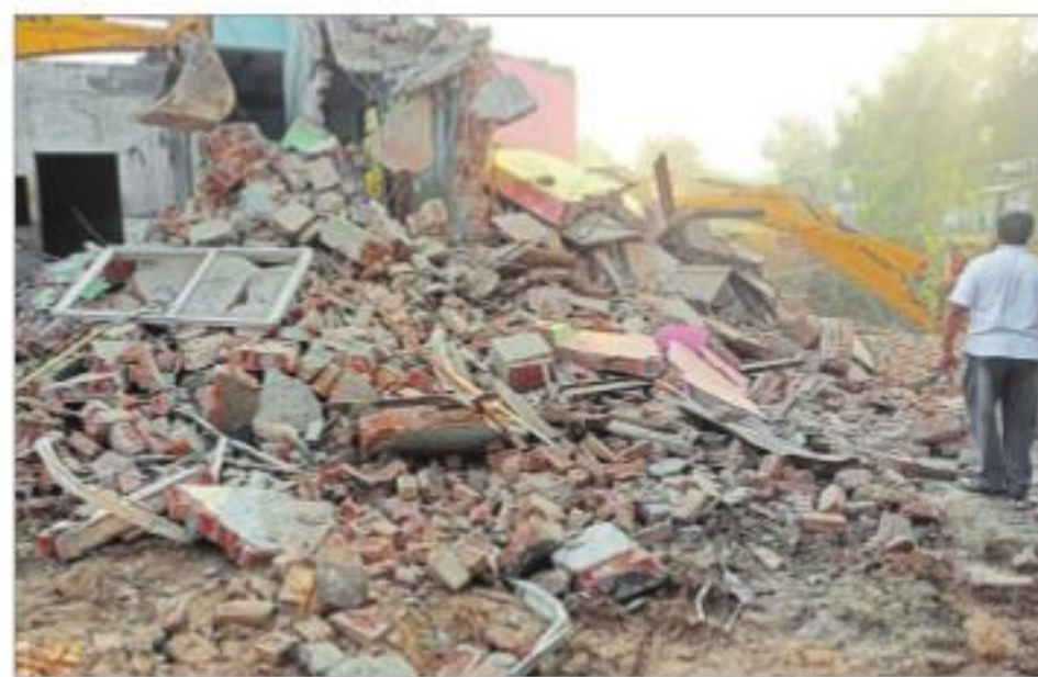
The illegal house of a drug smuggler being razed in Bhainsrawali.
